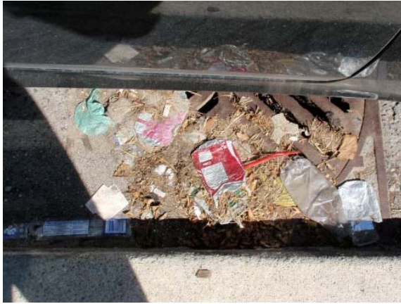
Figure 5.3 Accumulated Large Litter along a sewer drain and a curb
