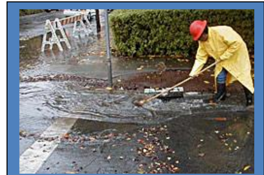
City employee works to clear clogged storm drain. Image: City of Palo Alto.
